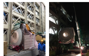
It took more than 7 hours to move the scanner into the room using a crane system (2014).
