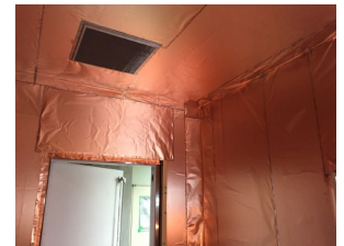
Magnetic shield Picture: 3T MRI room (at the time of under construction) in Shiga University of Medical Science
